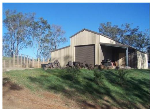
and then like a massive mechano set, joined the pieces and created a 11 x 12 metre, American Barn shed with a mezzanine floor. All of the iron cladding was second hand and bought from auction too. Two windows were purchase from recycling centres and the personal access door was off a job site which Graeme saved from being thrown out.
